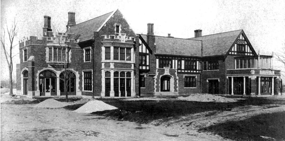
Mayslake Hall during construction, March, 1921. Photograph by Chicago Architectural Photographing Co.
